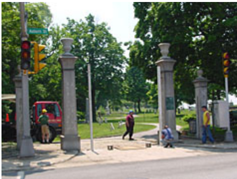
Removal of Currier Gate for Restoration
